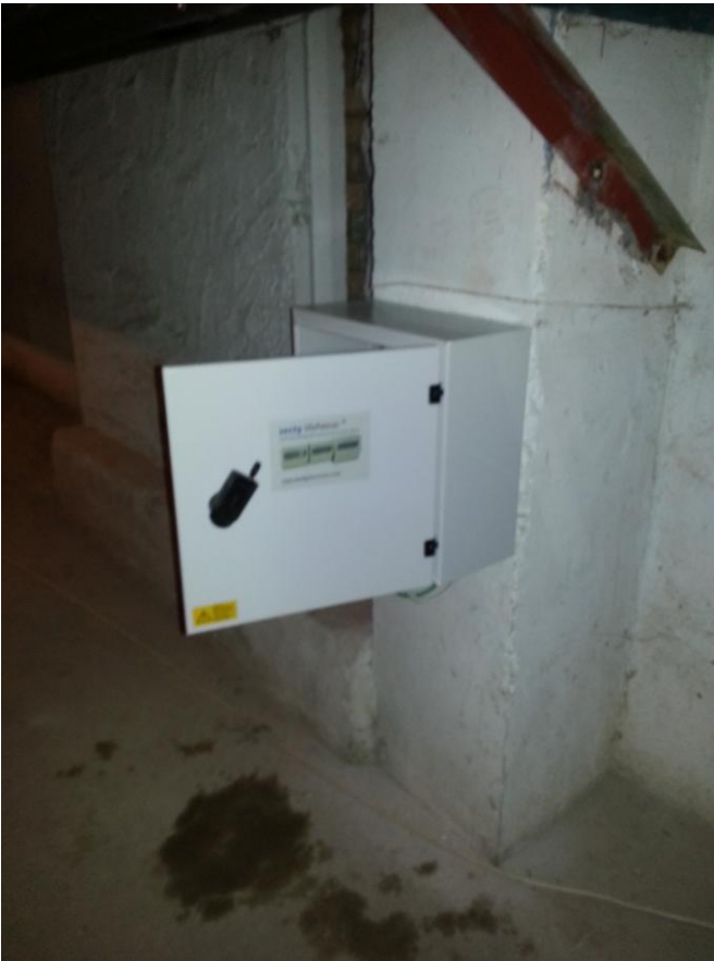
The siren cabinet was installed in a separate room.
