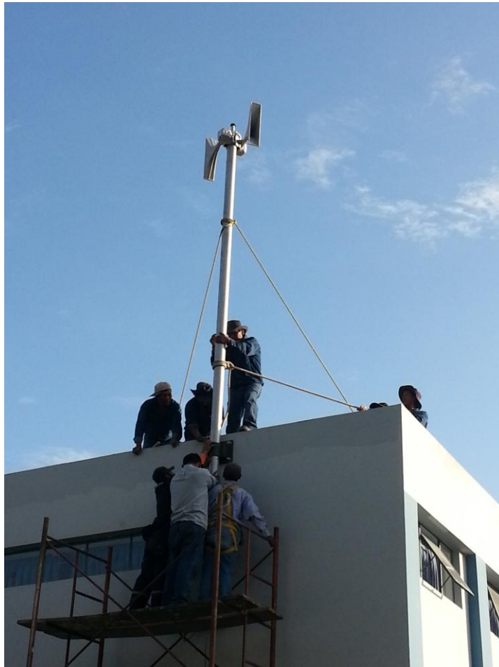
The siren mast is attached to the side wall of the building.
