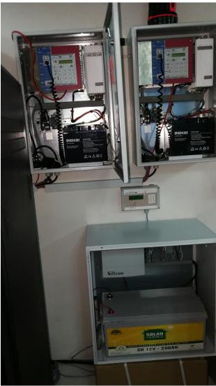
The secty central operator unit "TABD" and the siren cabinet with an additional UPS (200Ah) were installed in the control center. The earthquake system sends various messages from the 4 earthquake detectors to a computer and is saved there.
